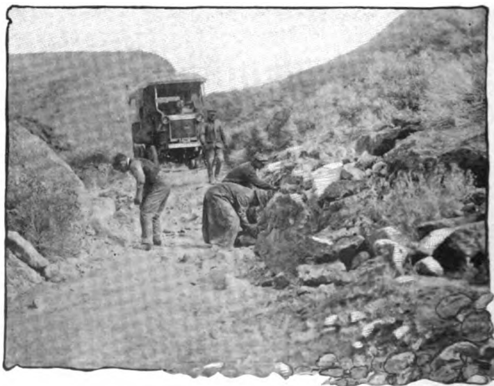
Blasting the rocks on a narrow mountain trail
